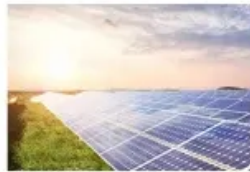
Energy Storage System
